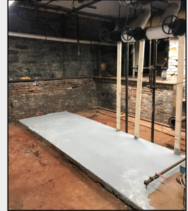
The concrete pad was repaired and painted in preparation.
