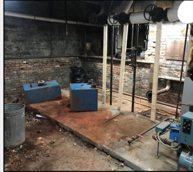
It was broken up and removed, leaving a giant mess.
