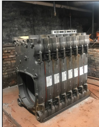
Assembly begins! Eight sections are bolted together and sealed.
