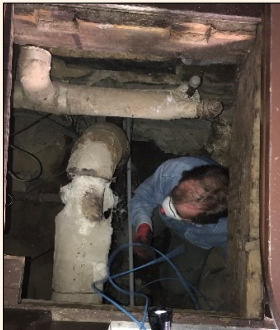
David pulls the cable into the underfloor cavity & routes it up a wall.
